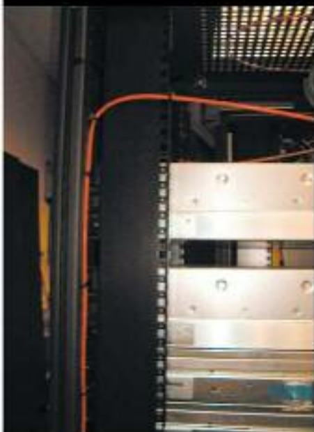
The red Firetrace Detection Tubing can be located in the rack in a manner that does not interfere with installation or maintenance of the equipment.
